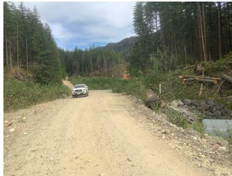
Running surface over culvert
